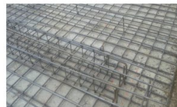
Steel Binding for Raft
