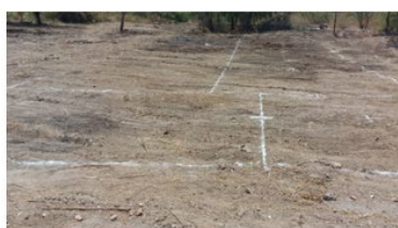
Survey and Layout at site
