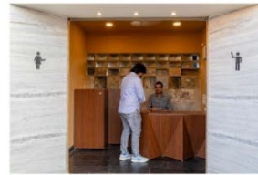
The lobby enables a transition space & can accommodate ATM & Tea Vending machine
