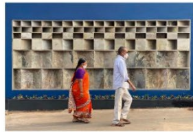
Porous facade made up of local natural Slate Stone from Telangana that enables Natural Light & Cross Ventilation throughout the day.
